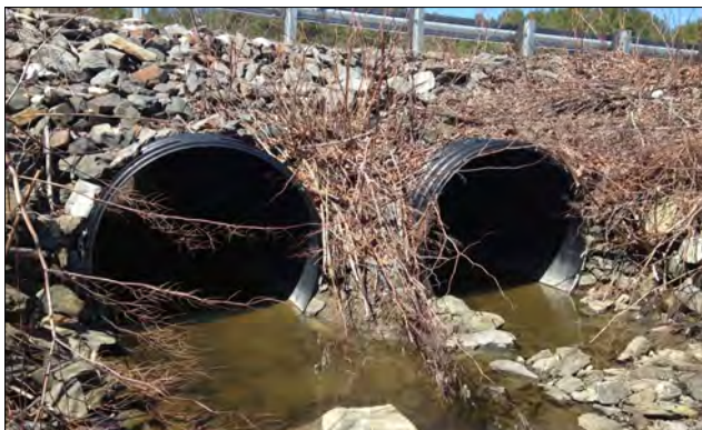
Figure 19: Payne Road culverts, 2015
