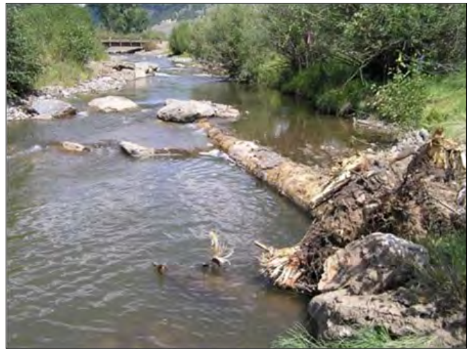
Figure 13: J-Hook log vane
