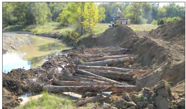
Figures 14 & 15: Wood toe structures
