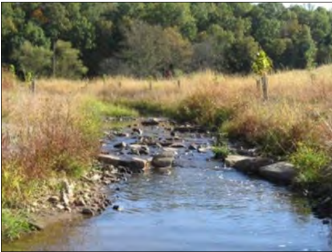
Figure 16: Constructed riffle
